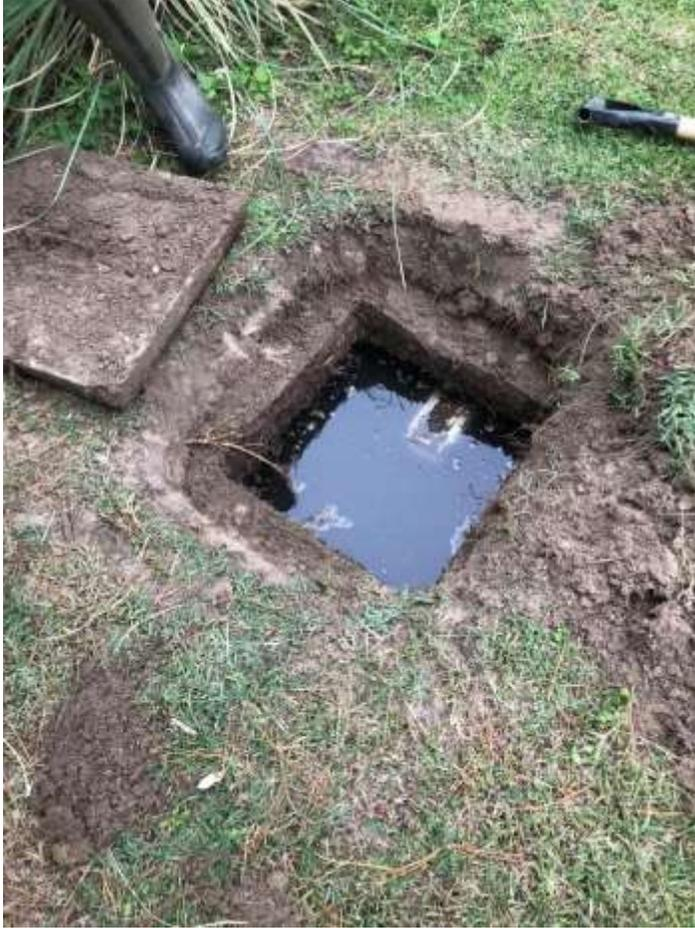
**Figure 3.11.** A septic tank in South Nags Head (RS) that was inundated by groundwater in November 2020.
